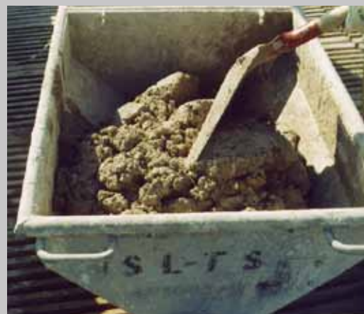
Grout in a mortar pump.
