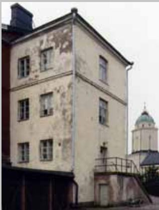
Stairwell A of the Bielke Bastion (C52) was built in 1847 as a latrine tower and converted to a stairwell in the 1890s. The slurry of the façade is cement mortar, apparently from the 1890s or 1913.
