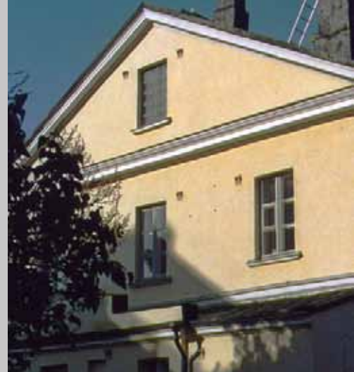
The lime and cement plaster of the south façade of the Old Pharmacy is carefully removed. The fragments of original surface plaster are left intact.
