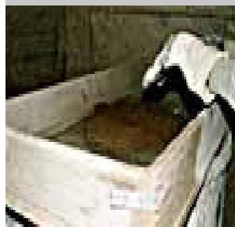
Screening of sand and mixing of mortar with a vertical-shaft mixer.
