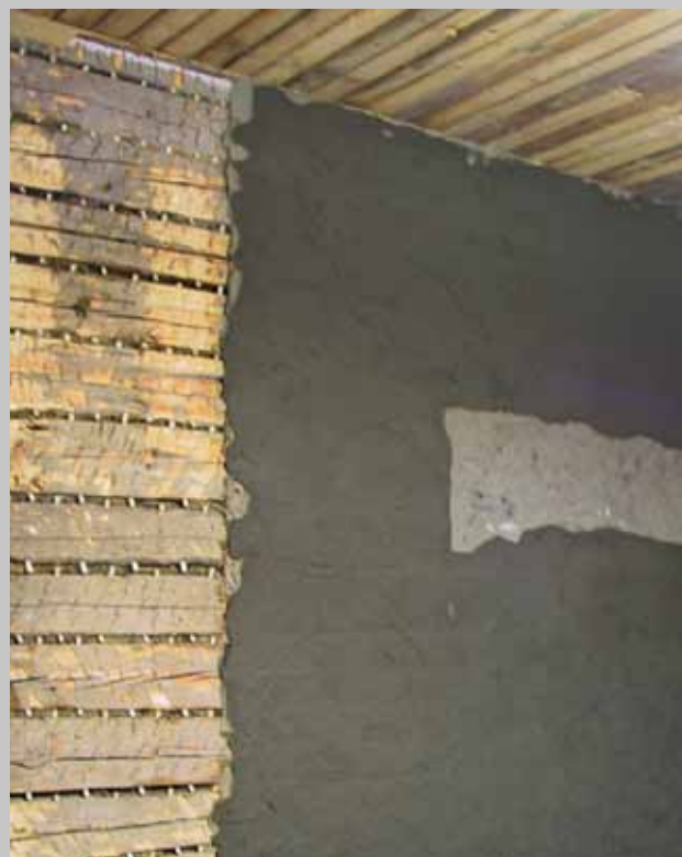
Old log wall with insertion pins and a new clay mortar plaster on top.
