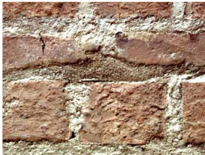
Parmu mortar used to repair the brick masonry of Häme castle was too hard for the old handmade bricks, resulting in breakage.
