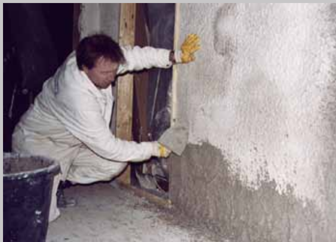
Plasterer Tommi Vilkanen coating the adhesion layer with a matured mortar...
