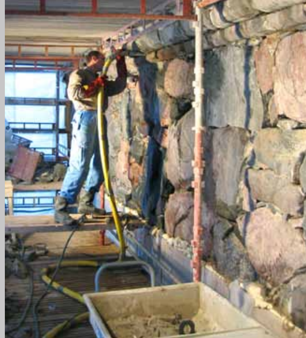
Holes in the masonry wall of Tenaille von Fersen are grouted with a mortar pump.
