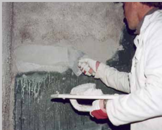
...and spreading the finishing coat exactly on the level of the old plastered and painted inner surface.
