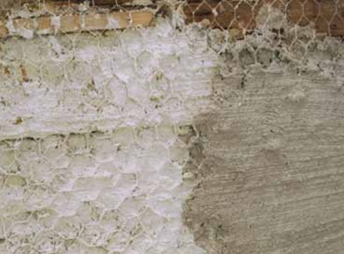
Old insertion pins, dowel rods, plastering mesh and adherence mortar on one of the log walls.
