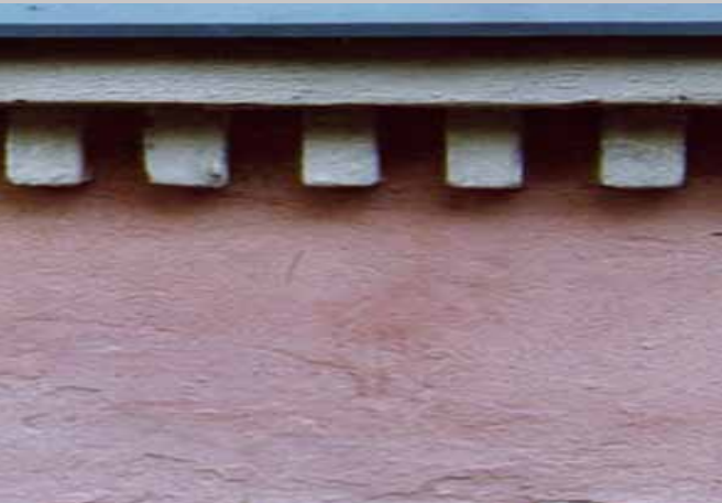
Original dentils under a window flashing of the Jetty Barracks (C1). They are moulded from a very cement-rich mortar, with aggregate making up only one third of the binder.
