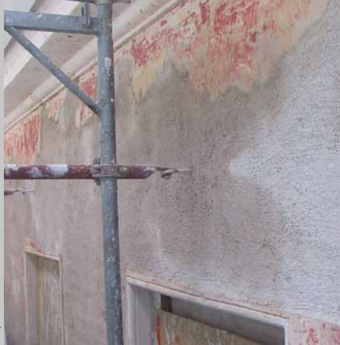
Finishing coat of the façade repaired with lime mortar.
