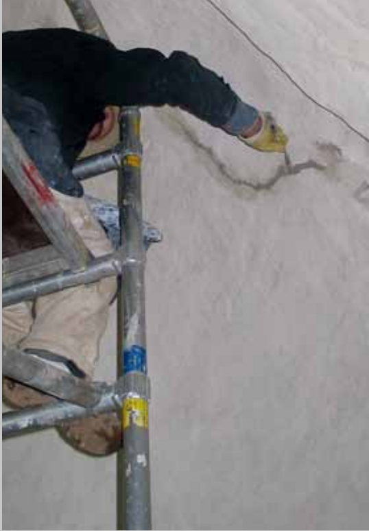
Fixing plaster from a scaffold.
