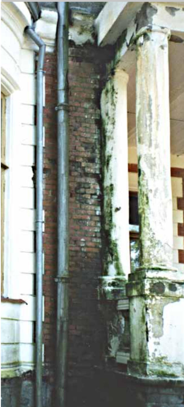
An effect of long-term moisture: moss has grown on the pillar surfaces.
