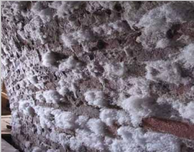
Crystallized salt on the surface of brick masonry. Cellar vault in the Tenaile von Fersen building of Suomenlinna.
