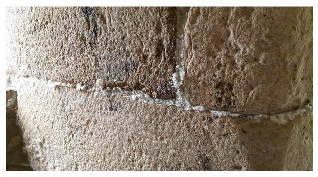
Figure 3: Sacrificial protection in practice - precipitation of soluble salts in mortar joints at Aydon Castle, Northumberland (18<sup>th</sup> century agricultural buildings).
