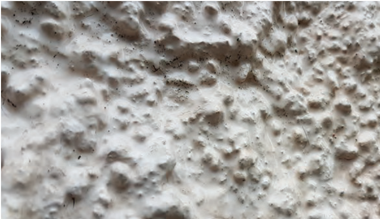
Fig. 9 Traditional lime harling, limewashed, becomes water-logged during heavy rainfall and forms a film of water on the outer surface to minimise water ingress.
