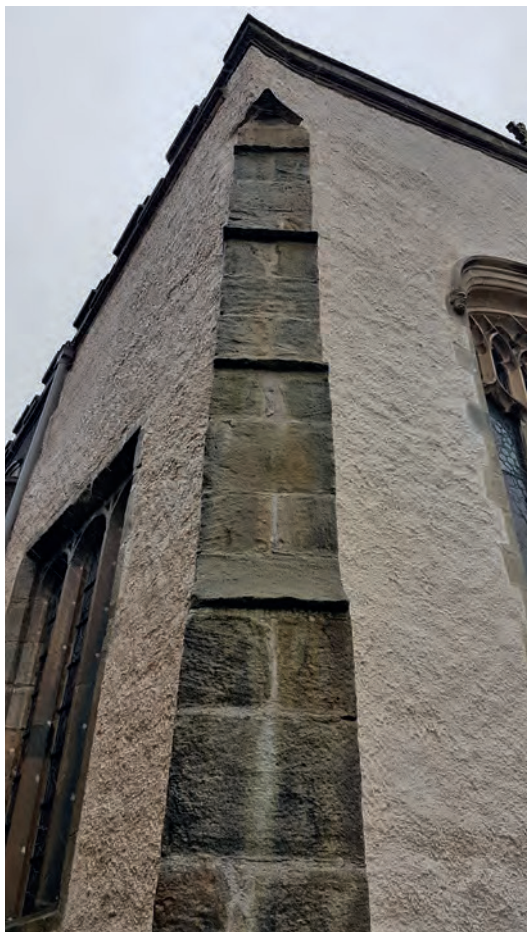
Fig. 10 Church of St Oswald, Warton, Lancashire. Traditional lime harling, limewashed, drying after wind-driven rain. The darkened side on the left is orientated towards the prevailing wind.
