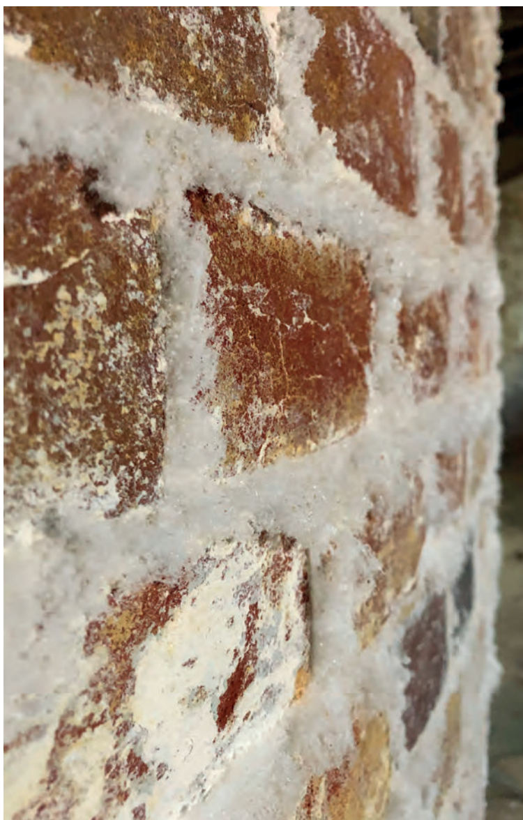
Fig. 12 Pronounced manifestation of sacrificial protection at work at Hurst Castle, Hampshire. The highly soluble salt load is being poulticed out of the coarse-pored brick substrate by the fine-pored traditional lime mortar (Credit: Kim Collins, Historic England).
