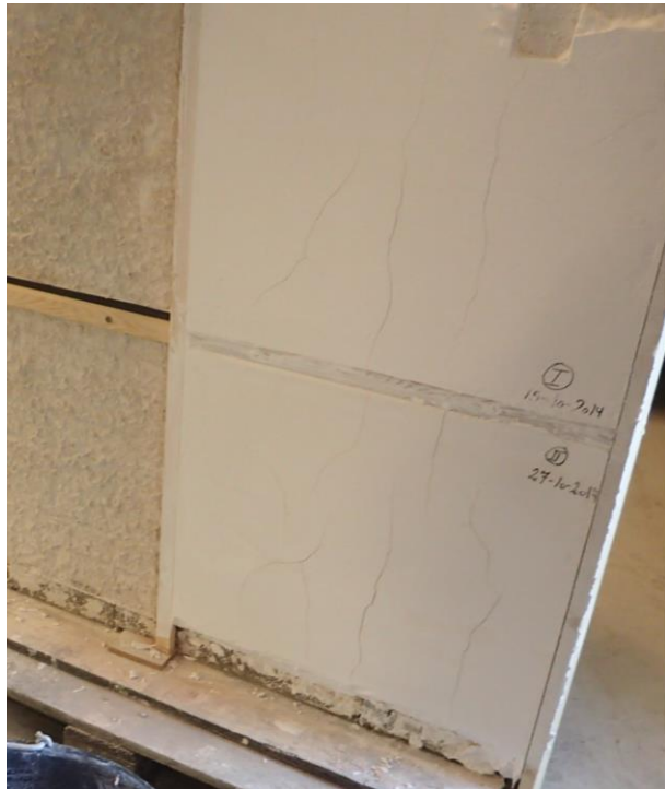
Figure 1. Rendered wall with \approx 20 mm insulating lime mortar.
