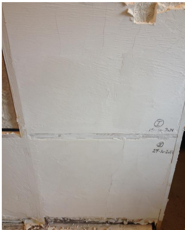
Figure 2. Rendered wall with \approx 20 mm insulating lime mortar and top coat to reduce appearance of shrinkage cracks.
