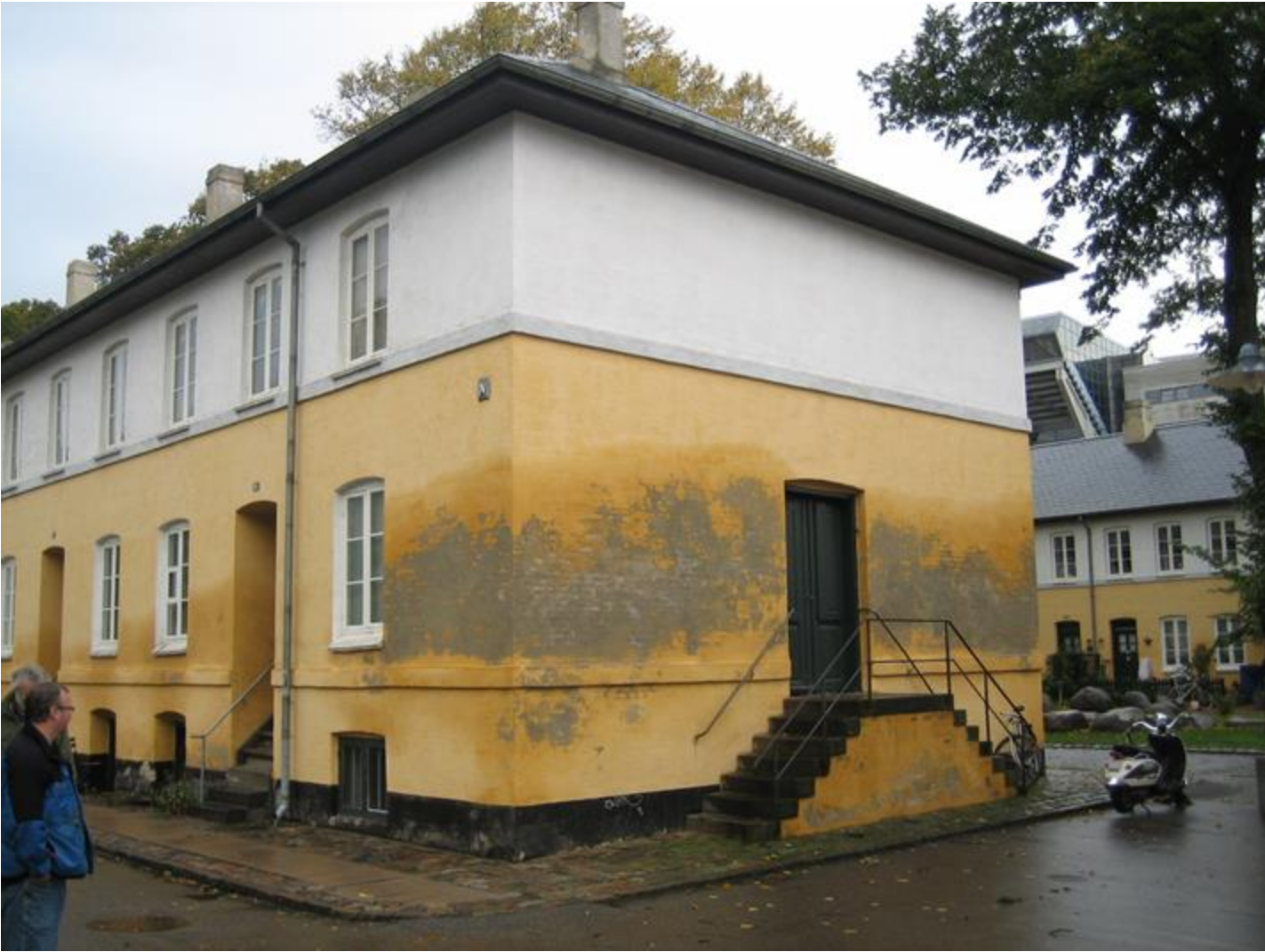
Brumleby, Copenhagen. Salt contaminated masonry. The wall is dry
